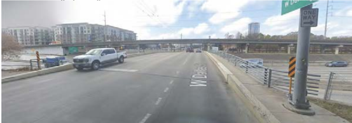
Figure 4: Current I-45 overpass at W. Dallas showing that it is not ADA-accessible, has no protected bike lane, has narrow sidewalks with no buffer from traffic, and no shade.
