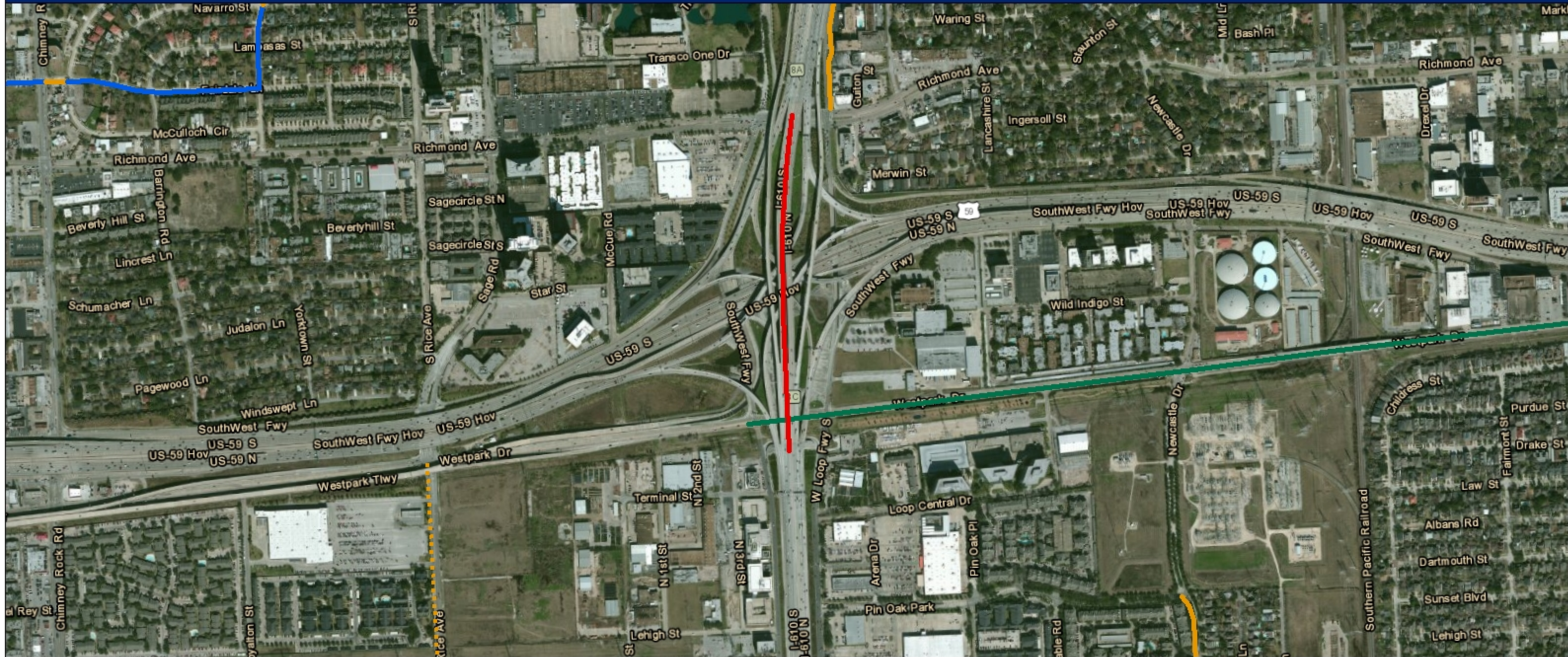
Description: Reconstruction of IH 610 Main Lane Bridge within the Interchange
