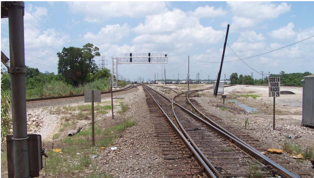
Photo 5-1: Mykawa Subdivision at New South Yard (looking north)
