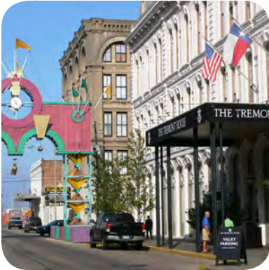
The City should take an expanded leadership role in promoting reinvestment and improvement Downtown and along key commercial and mixed use corridors.
