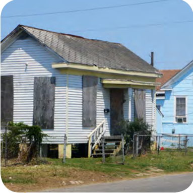
Citywide, deliberate demolition by neglect is a direct threat to the integrity of the historic fabric of the community.
