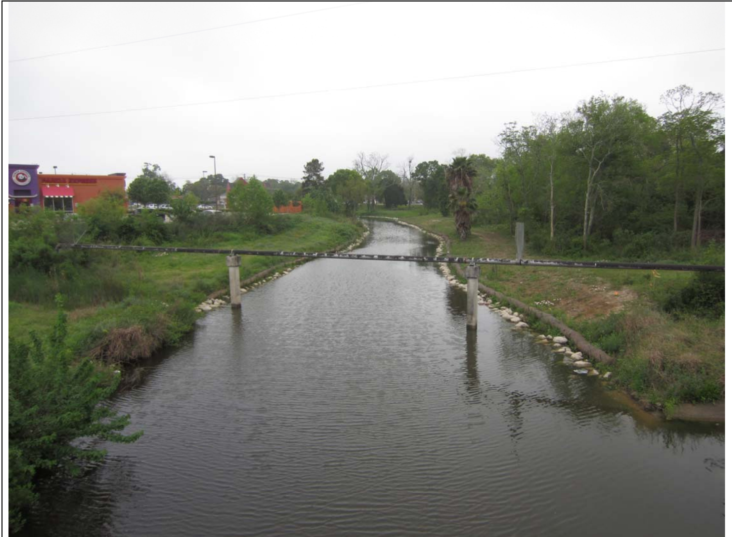
Robinson Bayou Upstream of the Proposed Bikeway/Pedestrian Bridge – Looking South from FM 270 Bridge.
