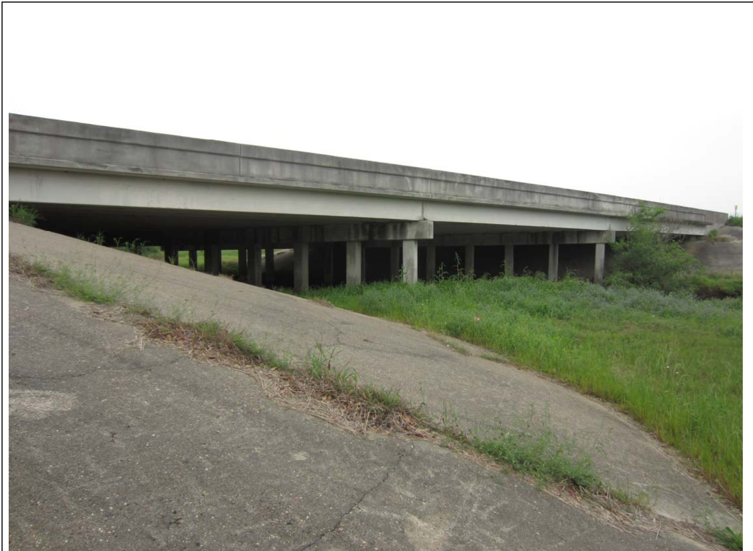
FM 270 Bridge Downstream Face – Looking Southwest.
