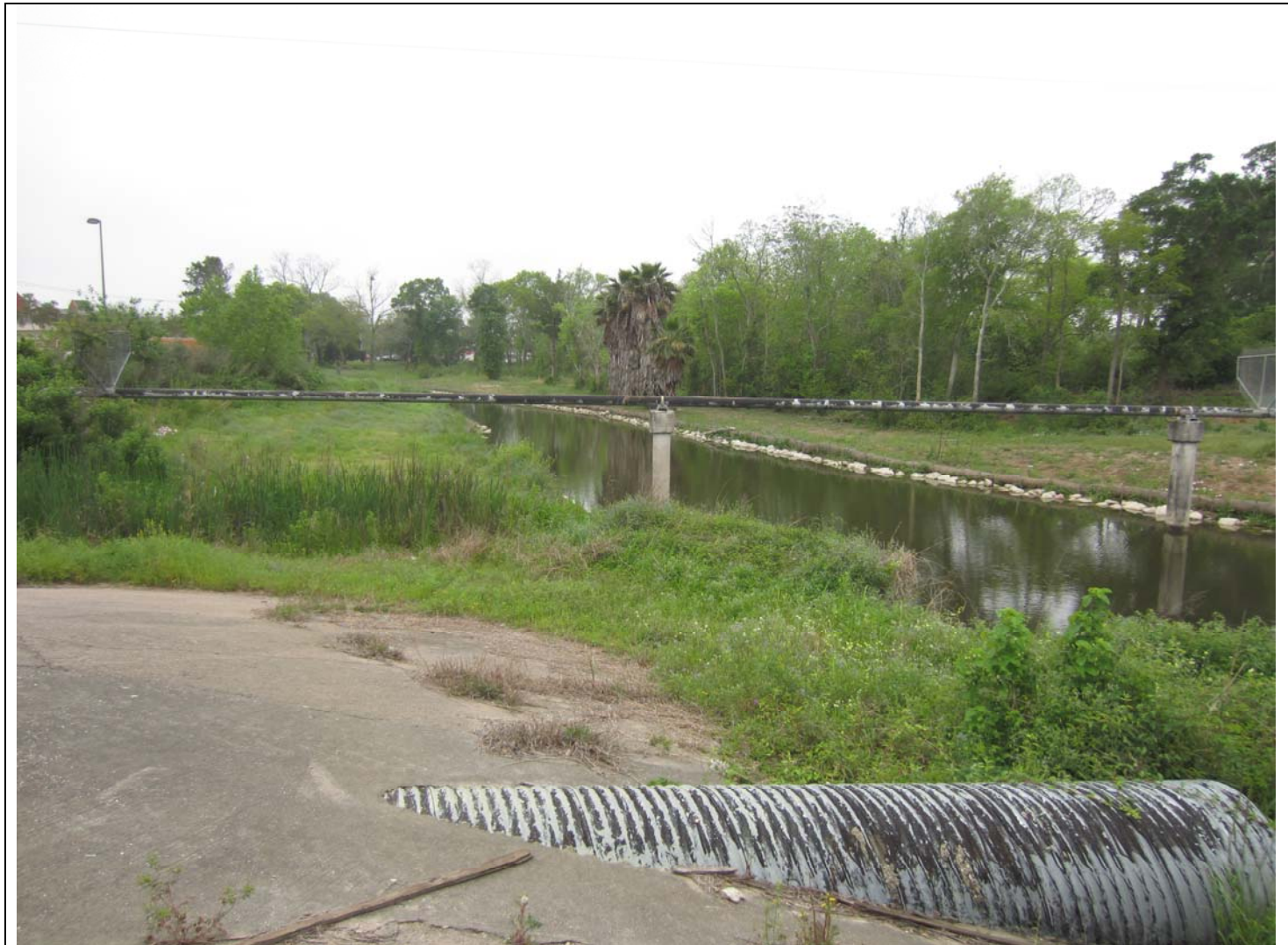
Robinson Bayou Upstream of the Proposed Bikeway/Pedestrian Bridge – Looking Southwest from the East Overbank.
