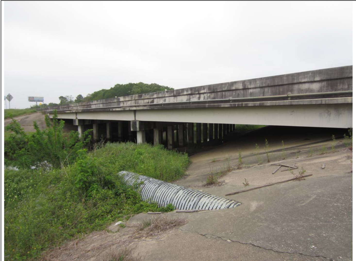
FM 270 Bridge Upstream Face – Looking Northwest.
