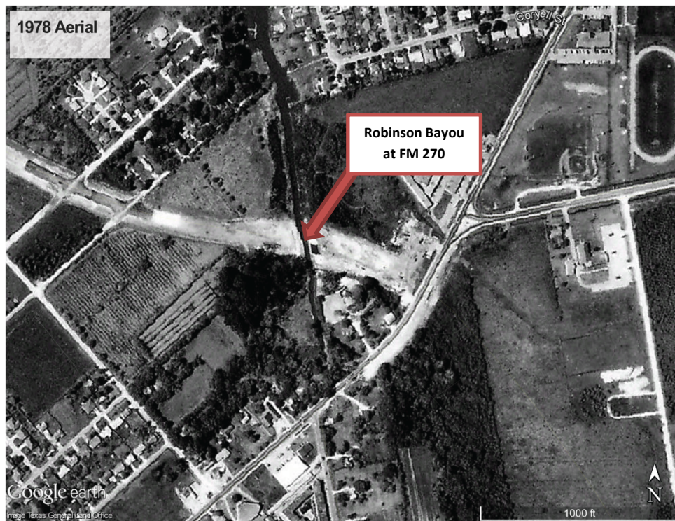
1978 Google Earth aerial photograph of Robinson Bayou at FM 270 crossing location
