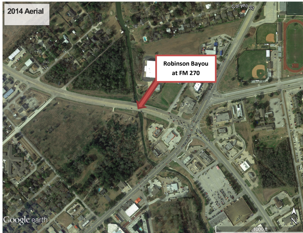
2014 Google Earth aerial photograph of Robinson Bayou at FM 270 crossing location
