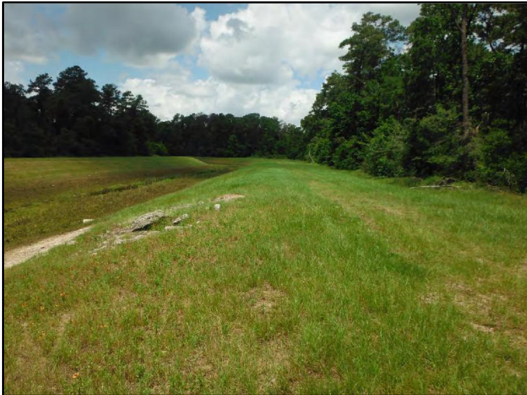
Figure 6. Overview of improved drainage (channelized bayou), view west
