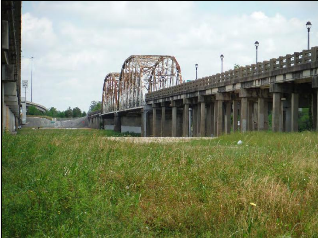
Figure 8. Overview of Bevil Jarrell State Highway 35 bridge, facing north.
