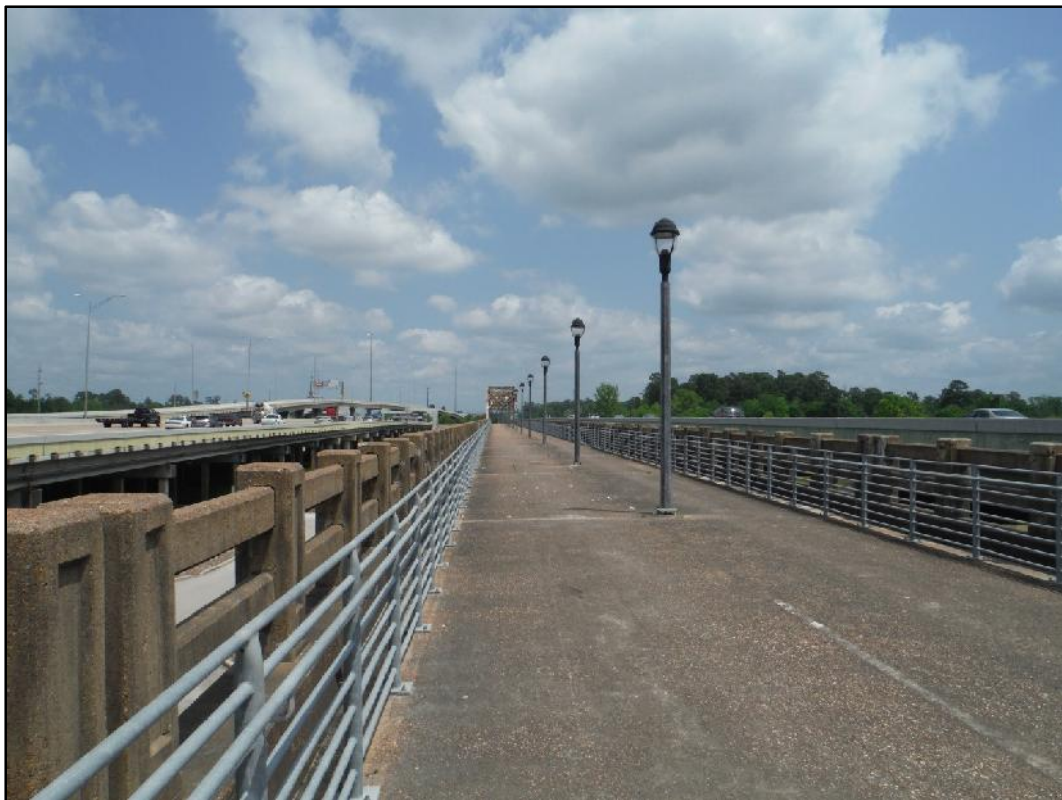
Figure 5. Overview of existing pedestrian bridge, facing north.
