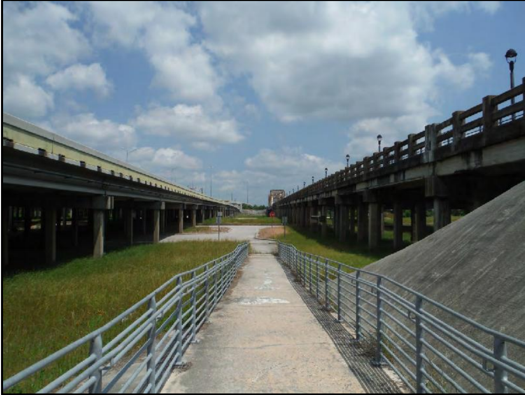
Figure 7. Existing concrete ramps, Bevil Jarrell State Highway 35 bridge, facing north.
