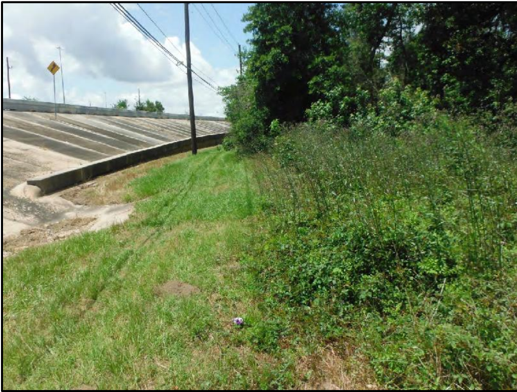
Figure 3. Overview of project alignment from midpoint, view south.
