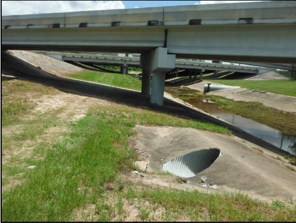
Figure 5. Highway 59, feeder road, and associated improvements to drainage, view east.
