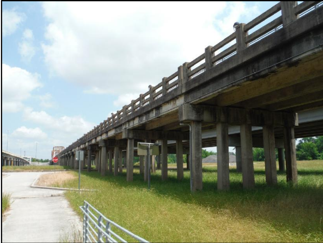
Figure 6. Overview of bridge showing supports, facing north.
