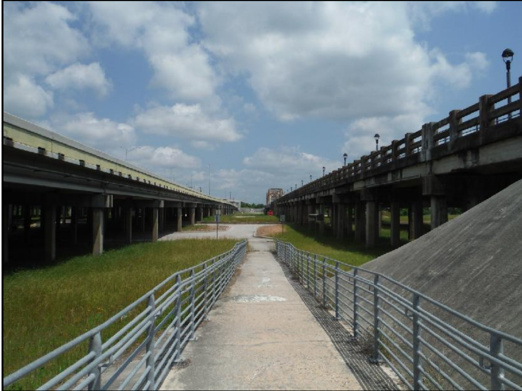
Figure 4. Overview of the existing ramp to bridge, facing north.
