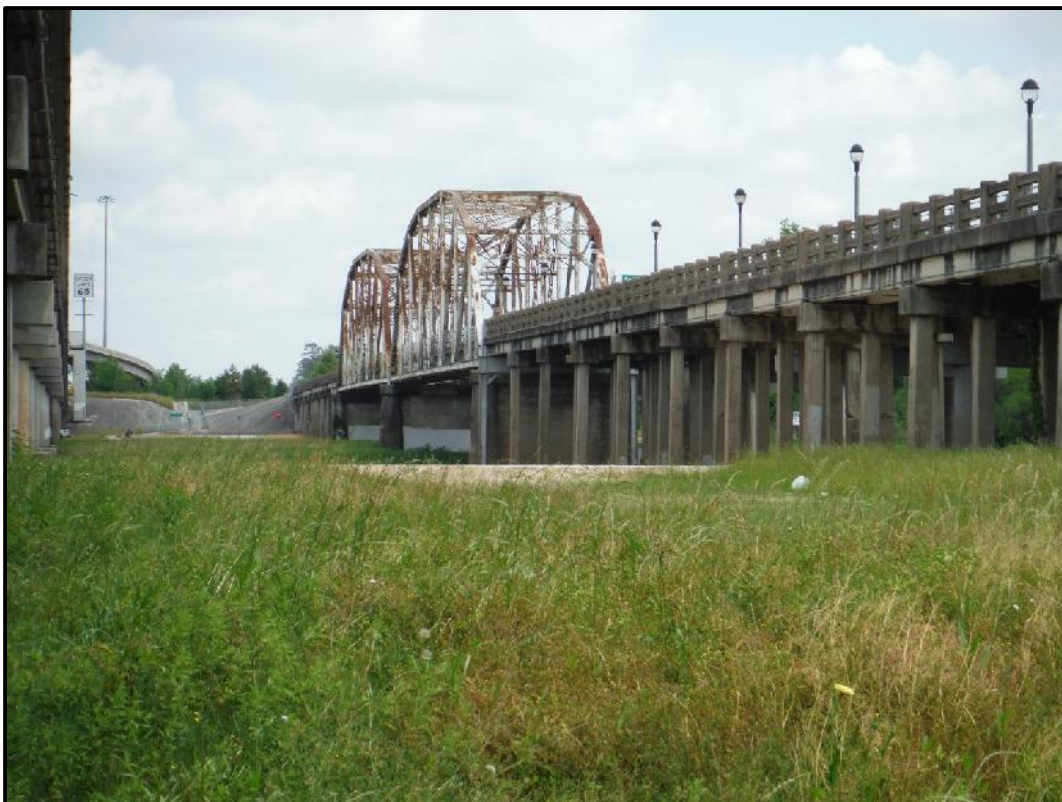
Figure 7. Overview of truss, facing north.
