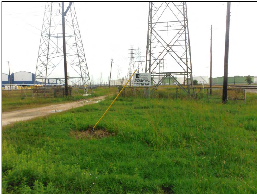
Facing east, this is a view of a portion of the transmission ROW located north of the PTRA railway.
