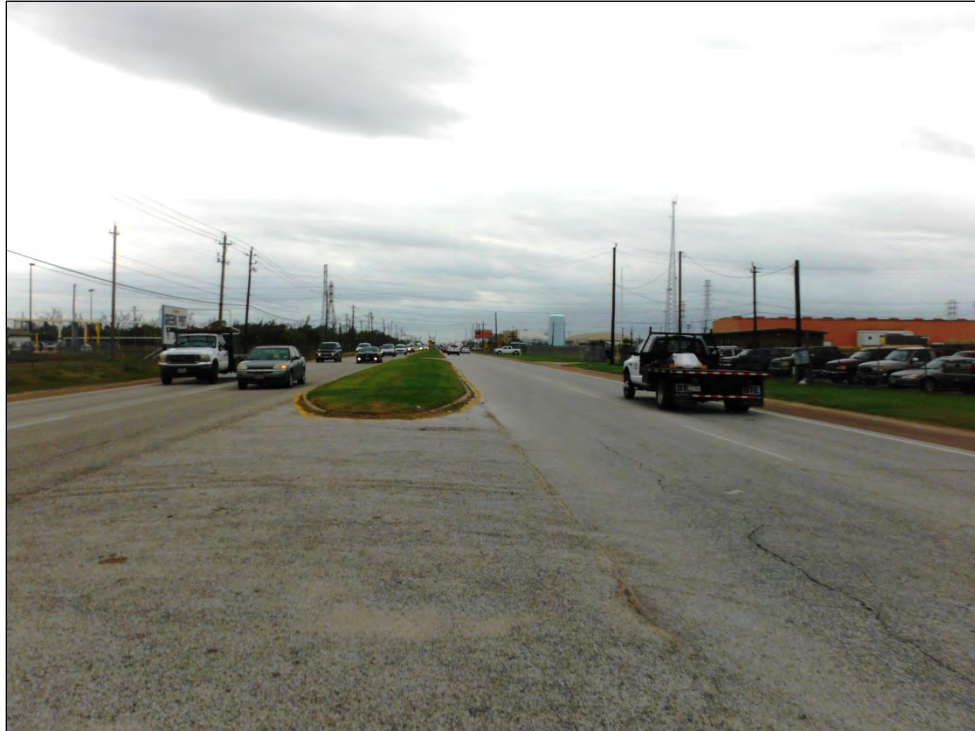
Facing south, this is a view of the northern section of the Federal Road ROW.
