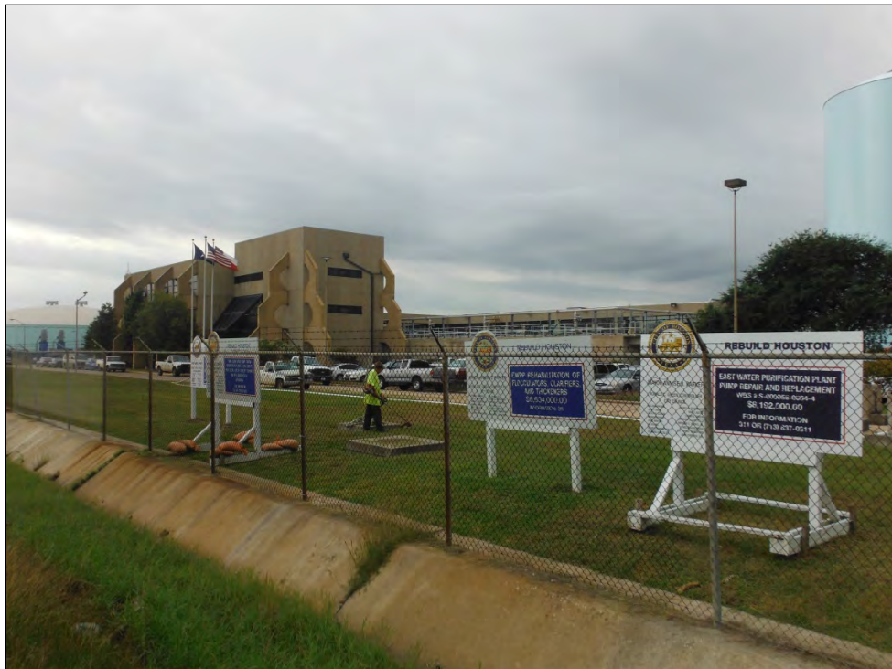
Facing south, this is a view of the East Purification Plant, adjacent to the proposed project area at 2300 Federal Road. A roadside ditch draining the proposed project area and adjacent properties is visible in the foreground.
