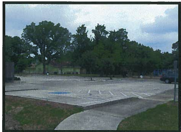
R. L. and Cora Johnson Community Center parking facilities
