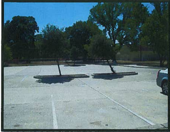
R. L. and Cora Johnson Community Center parking facilities
