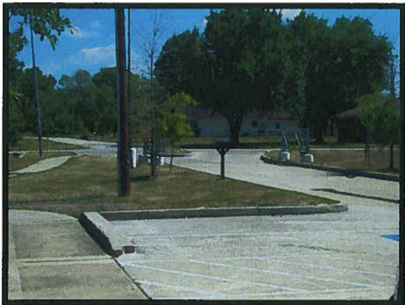
R. L. and Cora Johnson Community Center access entrance/driveway on Porto Rico
