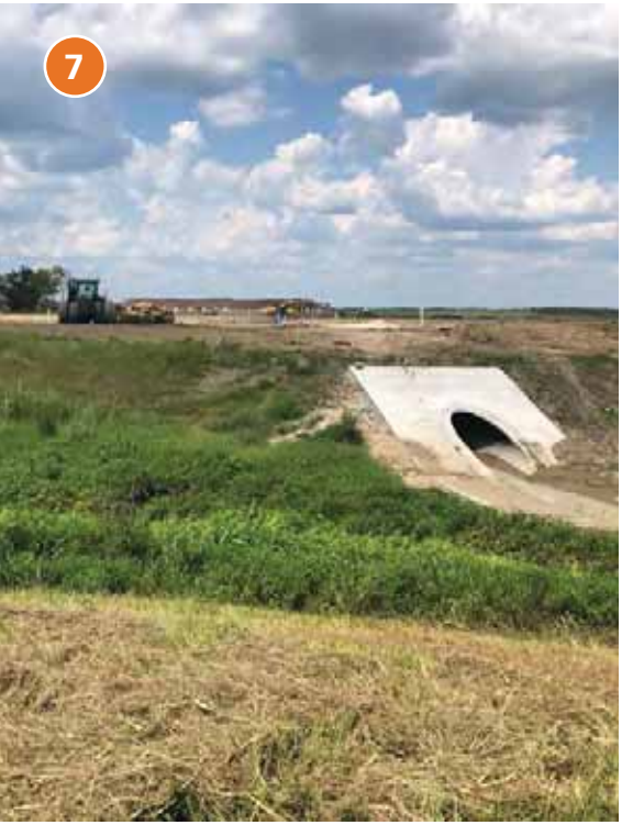
DRAINAGE OUTFALL AND NEW CONSTRUCTION This large outfall along the bayou will receive a significant portion of stormwater from the Champions Estates which is currently under construction.
