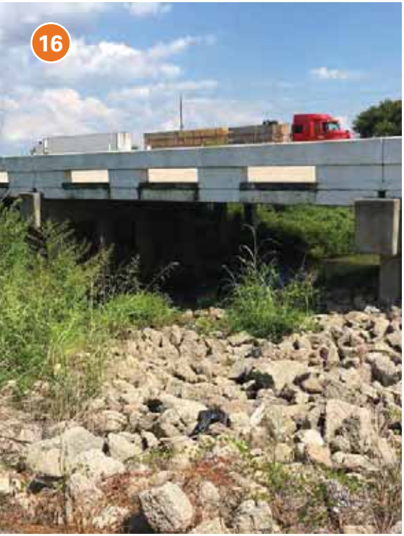
COTTON BAYOU AND I-10 The project site terminates at I-10 where the bayou flows under a bridge and a riprap exists to minimize erosion.
