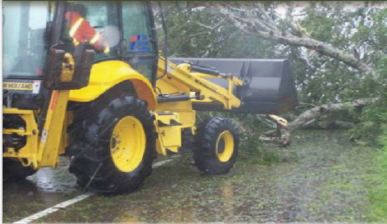
Emergency roadway clearing
