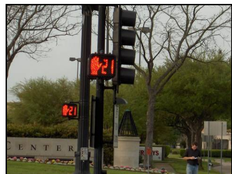
This pedestrian signal in Sugar Land features a timer to indicate how much crossing time remains.
