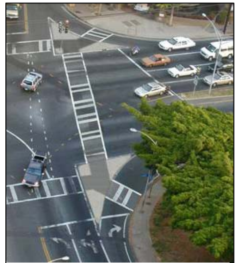
These sample channelized islands from Georgia Department of Transportation illustrate the system of crosswalks.
