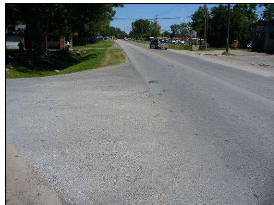
Gulf Bank Road West of Airline Drive, looking East
