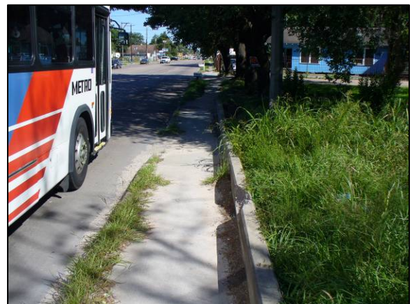
These sidewalks on Airline Drive near Hill Road (above) and Mount Houston Road (below) are in fair to good condition, but pedestrian space is constricted, and the ramp and crosswalk do not meet current standards.
