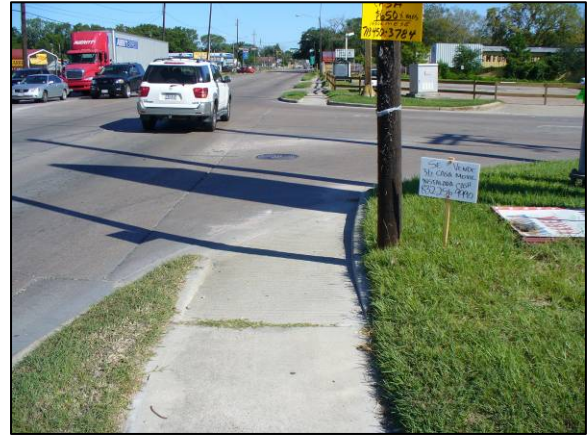
These sidewalks on Airline Drive near Hill Road (above) and Mount Houston Road (below) are in fair to good condition, but pedestrian space is constricted, and the ramp and crosswalk do not meet current standards.
