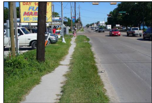
This sidewalk on Airline Drive near Mount Houston Road is in good condition, although it is too narrow by current standards, and grass covers the edges.
