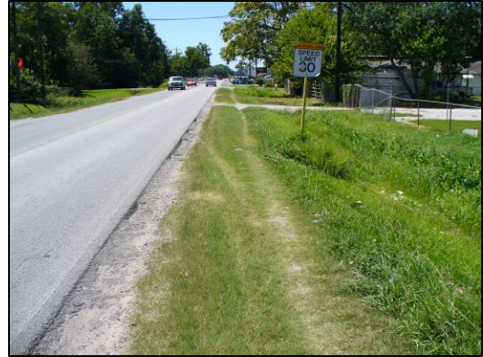
Gulf Bank Road West of Airline Drive, looking West
