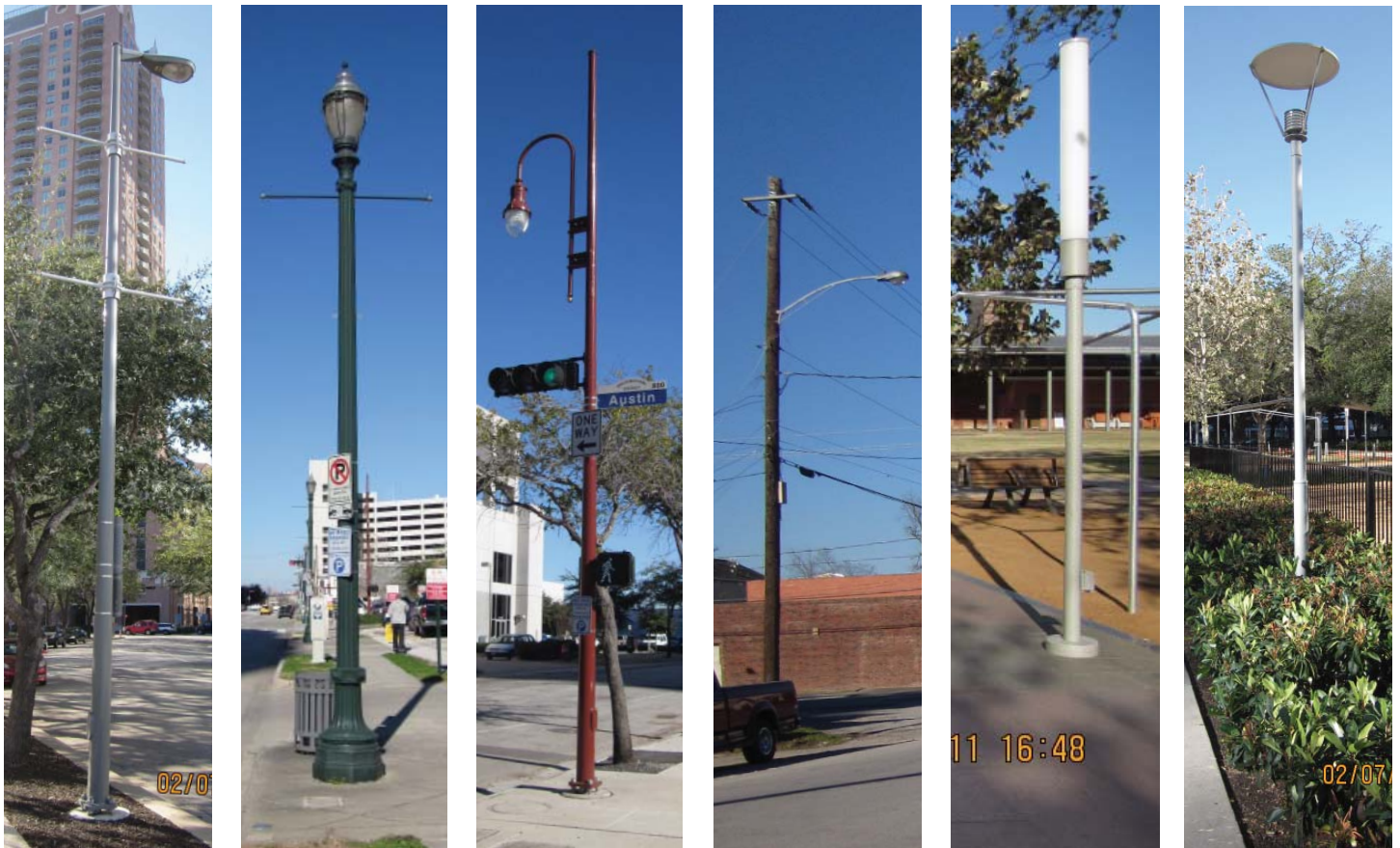
From Left to Right 1 Vehicular Street Lighting: Standard Downtown, 2 Vehicular Street Lighting: Historic District, 3 Vehicular Street Lighting: Ball Park District, 4 Vehicular Street Lighting: Utility Pole Mounted, 5 Pedestrian Lighting: Discovery Green, 6 Pedestrian Lighting: Discovery Green
