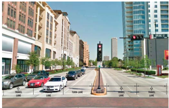
Photo Raised median with pedestrian safe-zone
