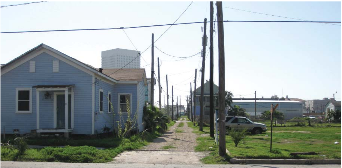
Photos Overhead utilities in the study area
