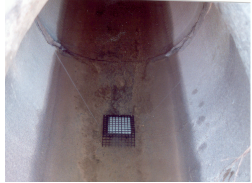
Figure 14: OB device deployed in storm drain.
