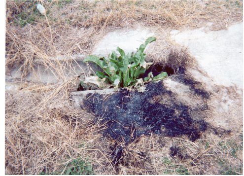
Figure 8. Oil dumped at a storm drain outfall.
