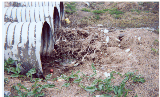
Figure 6. Trash and debris washed out of the storm drain.
