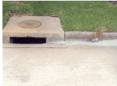
Figure 9. Paint stained concrete.
