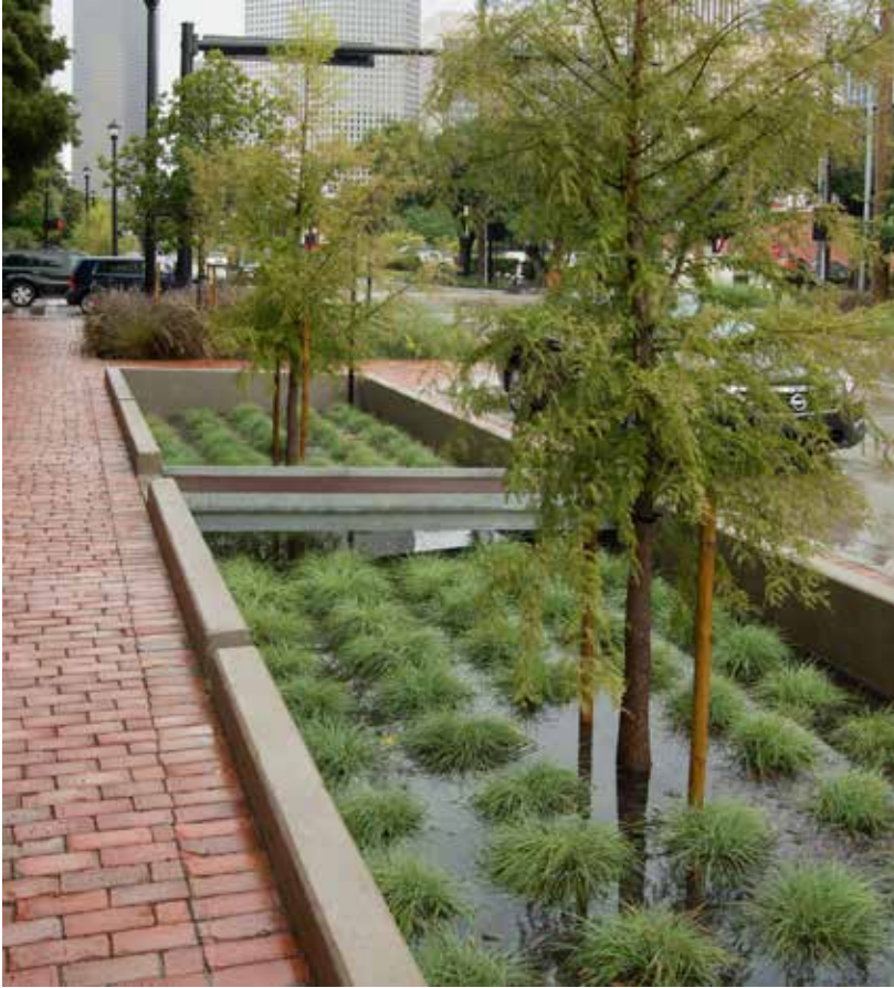
Rain gardens along Bagby Street in Houston filter and clean urban runoff before it flows to the adjacent Buffalo Bayou.
