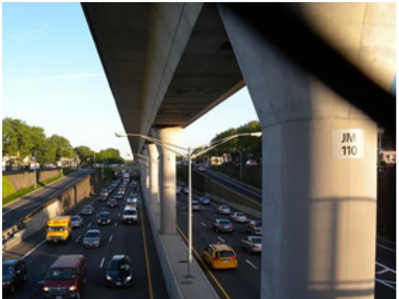
Figure E3.17: EXAMPLE OF ELEVATED TRANSITWAY ALONG FREEWAY CENTERLINE
