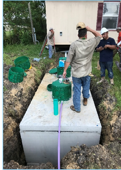
Figure 4. Septic tank replacement
