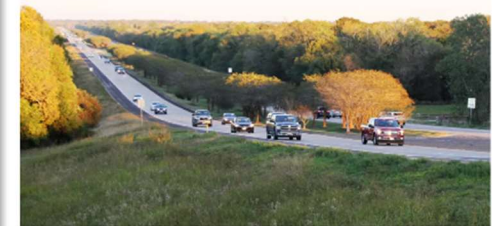
US 90 from El Paso to Dayton is a major thoroughfare for east-west traffic. In recent years, due to growth and other factors, it is not uncommon to see westbound traffic backed up in the Tishy flow bottom, causing frustration and safety concerns.
