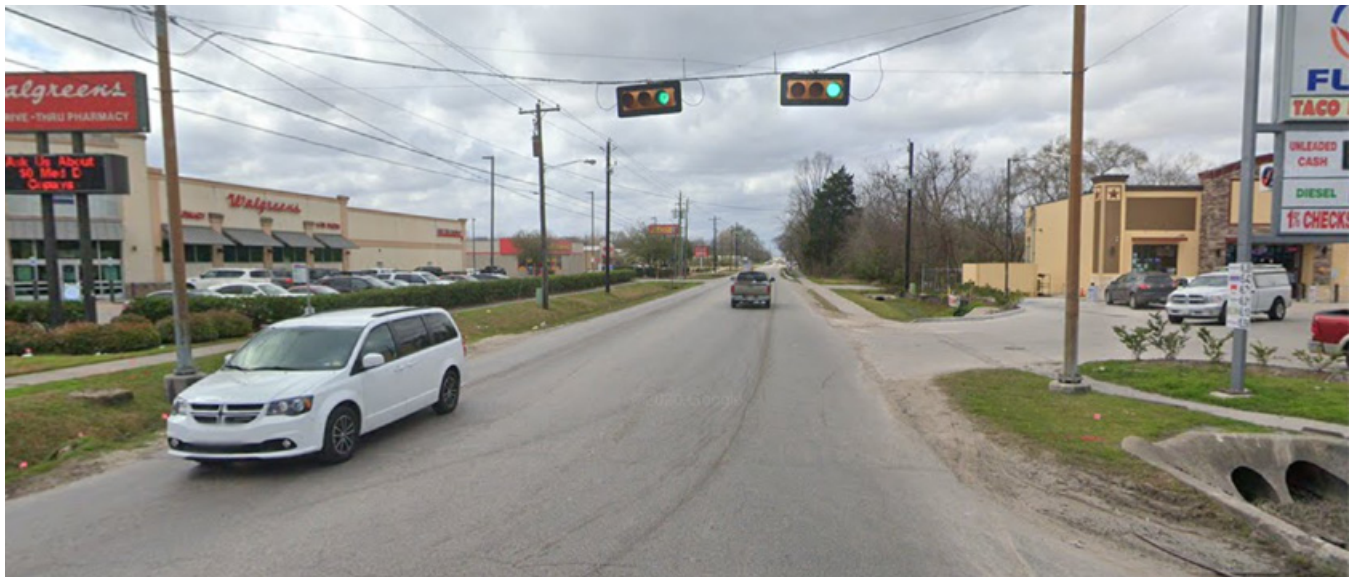
Signalized Intersections with moderate-to-high vehicular volumes but without dedicated, protected left turn phases, such as at the intersection of Aldine Mail Route at Aldine Westfield Road, limit total intersection capacity while also increasing the risk of collision with oncoming vehicles and crossing vulnerable road users. A Harris County CIP project is currently addressing this intersection. Source: Traffic Engineers Incorporated.
