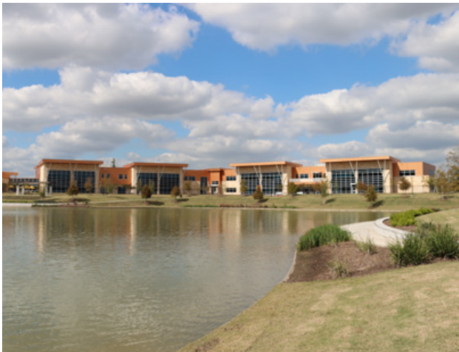
Detention basin at the Town Center development. Source: Traffic Engineers Incorporated.
