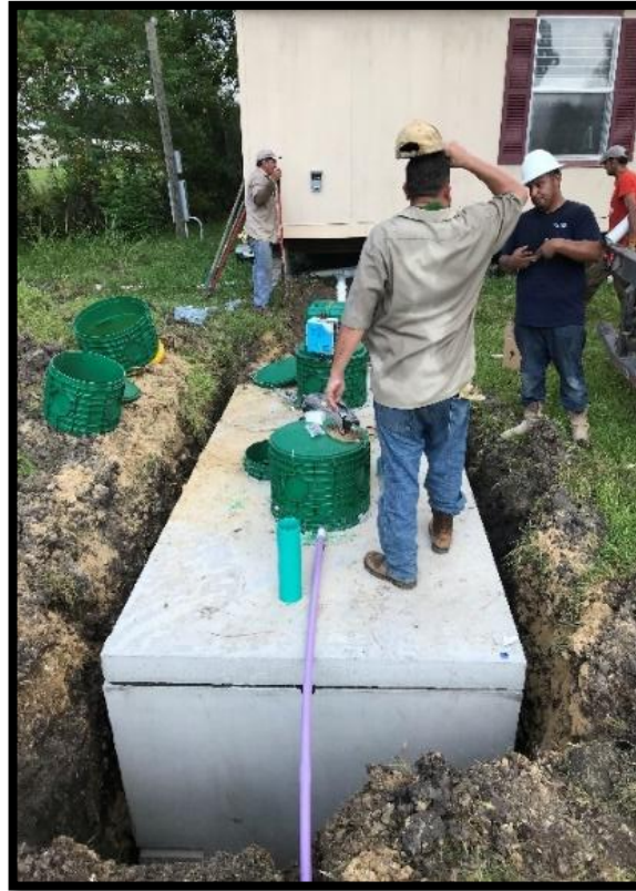
Figure 7. Septic tank replacement
