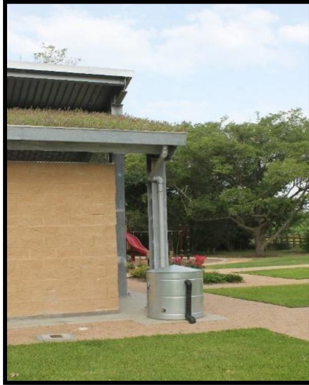
Figure 6. Green roof and rain barrel at Ghirardi Watersmart Park, League City, TX Walker County Addressing Onsite Sewage Facility (OSSF) Compliance (2015 Annual Report)
