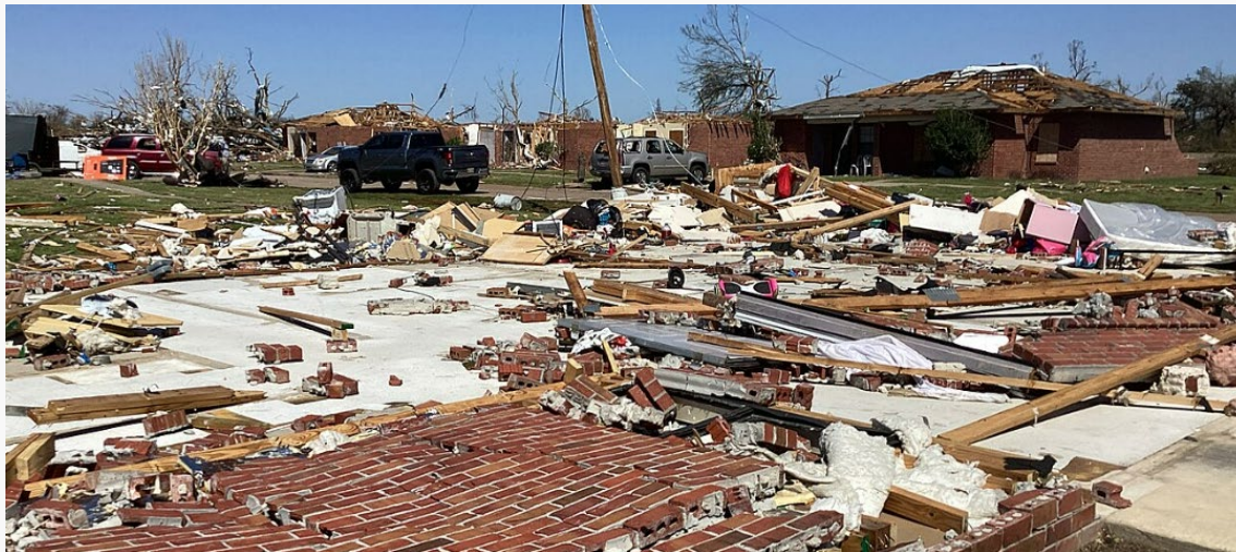
EF4 Tornado Damage to a Duplex (NWS Picture)
