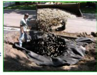
rock infiltration sump under the garden. This "rock baggie" helps water infiltrate quickly.
