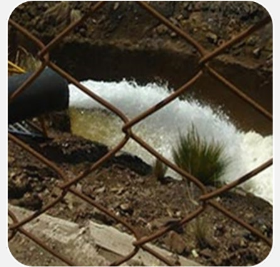
Polluted stormwater is deposited directly into streams without being treated
