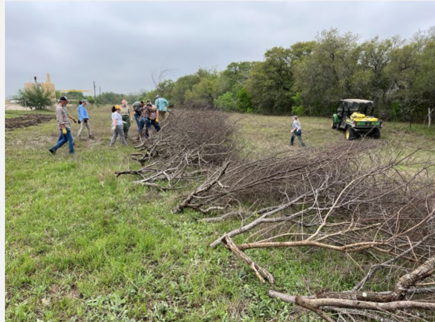
Above: Repurposed brush to slow runoff and catch sediment
