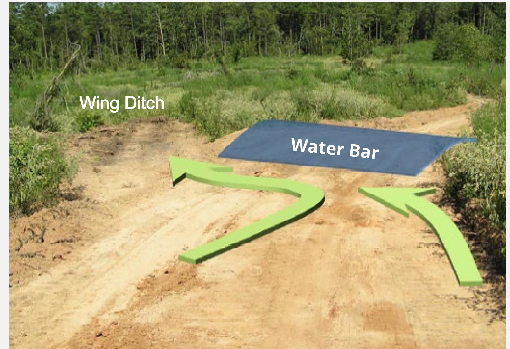
Properly constructed wing ditch with water bar directing flow.
