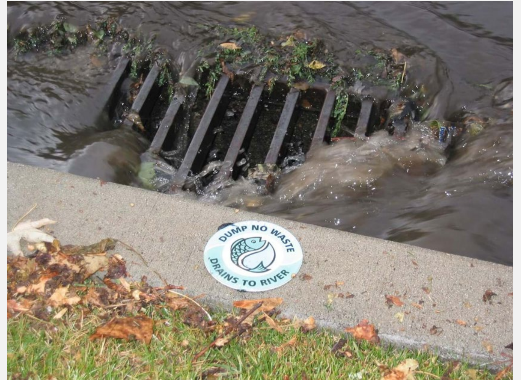
An educational sticker next to a suburban stormwater drain.
