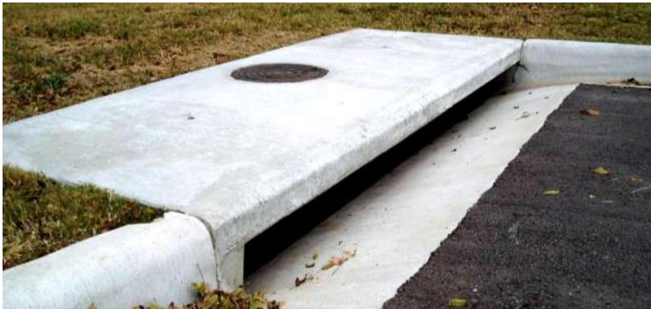
Figure 7.2. Storm drain in Kyle adjacent to Steeplechase Park. Stormwater engineering analyses are an important initial part of the urban management strategy.
