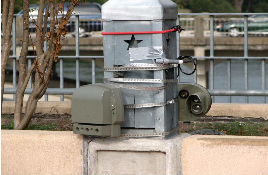
(Equipment shown in a temporary controlled testing configuration)
