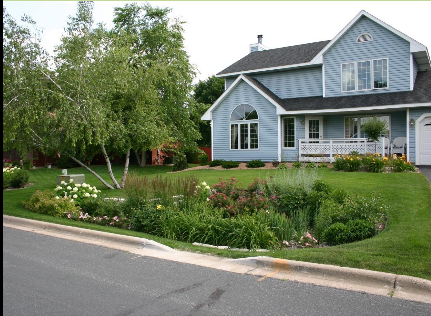
Raingarden (Bioretention Cells)
