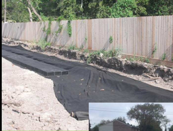
Alley Underdrain Construction
