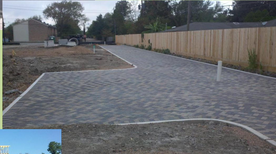
Completed Paver Alley
