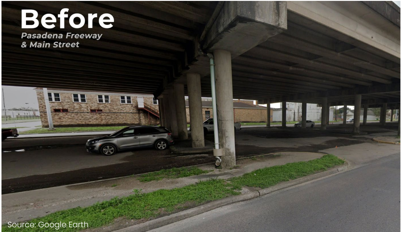
Figure 66: Existing Parking Conditions Under SH 225
