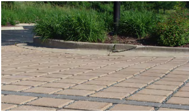
Porous pavers. Source: Center for Neighborhood Technology
