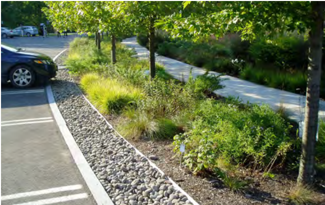
Example of Low Impact Development that infiltrates stormwater flowing off a parking lot. Source: Tomkins County
