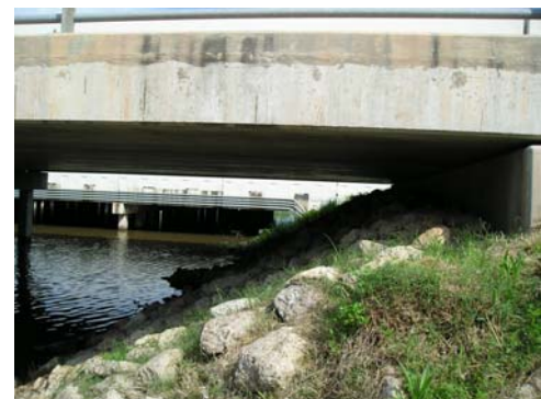
The clearance under this bridge appears too low to accommodate a pedestrian underpass.
