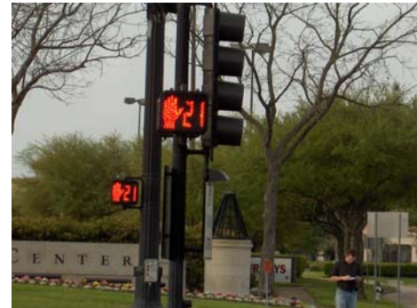
This pedestrian signal at SH 6 and Town Center Boulevard features a timer to indicate how much crossing time remains.
