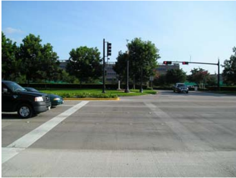
Unlike most locations along SH 6, the Kensington Drive traffic signal does not have crosswalks.
