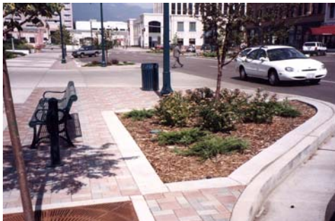
Curb extension with driveway, Colorado Springs CO. The design provides a place for drivers to wait for a gap in traffic without blocking the sidewalk.
