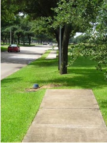
A short section of missing sidewalk on First Colony Boulevard.
