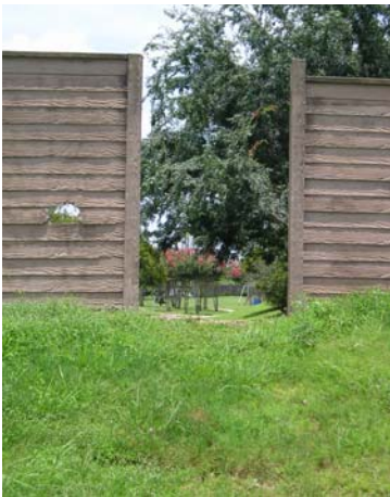
Pedestrians are able to pass through this fence opening behind Lowe's.
