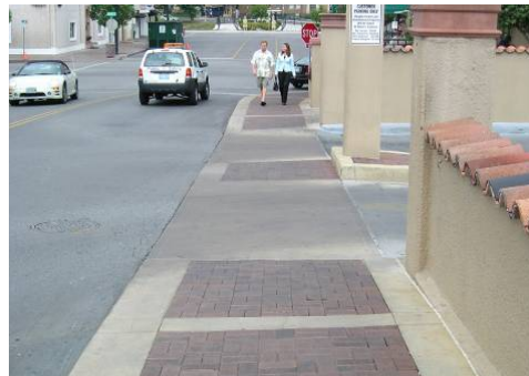
These two sidewalks share the same problem. The sidewalk visually breaks for the driveway and there is nothing to indicate to drivers they are crossing a pedestrian route. (Charleston WV at left; Kansas City MO at right)
