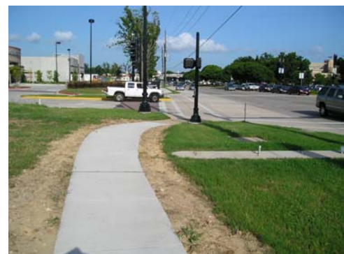
The curve in this sidewalk may lead blind or visually-impaired pedestrians into the intersection at the wrong angle.
