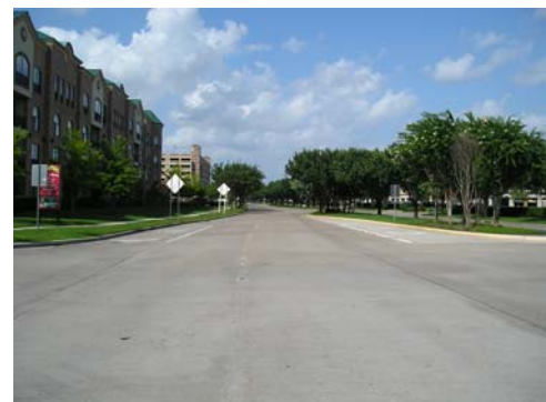
The lack of crosswalks at Lone Star Drive makes it difficult to know the appropriate location to cross.
