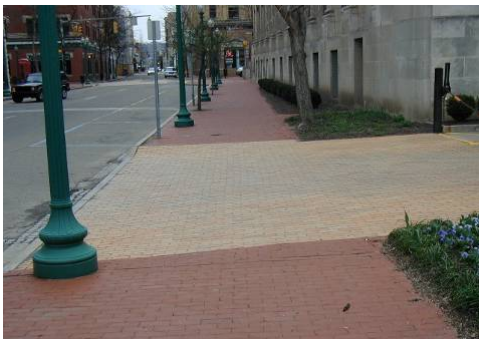
These two sidewalks share the same problem. The sidewalk visually breaks for the driveway and there is nothing to indicate to drivers they are crossing a pedestrian route. (Charleston WV at left; Kansas City MO at right)
