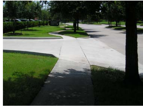
The older driveway at top is depressed to street level, requiring curb ramps and allowing motorists to enter at higher speeds. The newer driveway below is level with the sidewalk.
