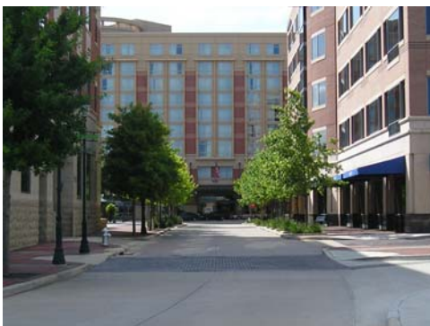
Pedestrians may suddenly appear from behind City Hall on the left. This is Plaza Drive between City Hall and the Texas Garage.
