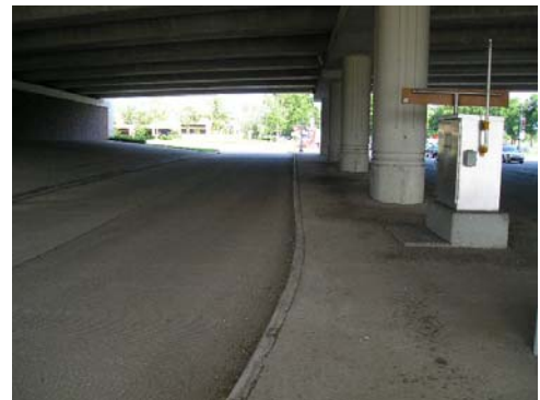
Railings and lighting would make the US 59 underpass less intimidating to pedestrians.
