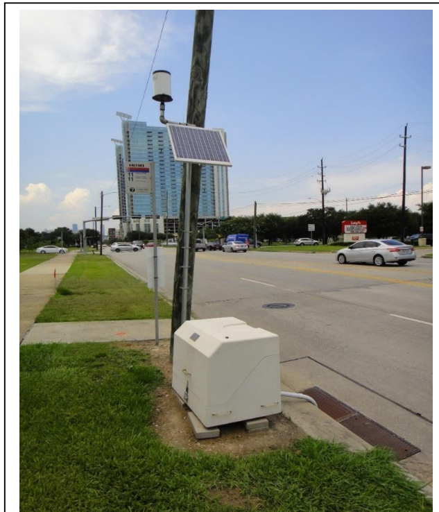
Figure 9. The City of Houston Urban Street Rebuild on Almeda Rd. automated sampler for the BPA LID BMP preconstruction monitoring project.
