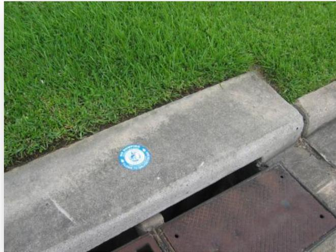
**Figure 106 –Stormwater drain with marker**
