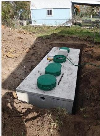
**Figure 60 – OSSF being installed**
