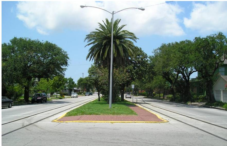
This median nose on 25<sup>th</sup> Street (Rosenberg) illustrates the refuge area (paved in red brick). The crosswalks connect to either end of this refuge area, but they are difficult to see and should be replaced with new thermoplastic markings.
