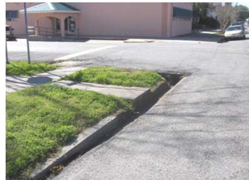
This corner of Broadway and 19<sup>th</sup> is a good example of an intersection not meeting ADA. There are no curb ramps at all, and the gutter is very deep, producing a tripping hazard.
