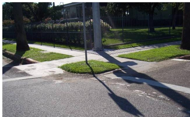
These sidewalks transition directly into the street, without ramps or detectable edge markings.
