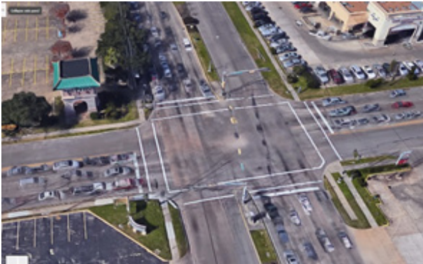
Boone Road and Bellaire Boulevard where there is higher walking demand represents an opportunity to improve safety and add walk infrastructure
