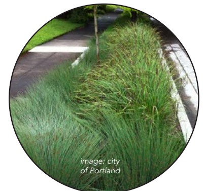
A thriving roadside bioretention swale featuring a well-composed naturalized planting mix.
