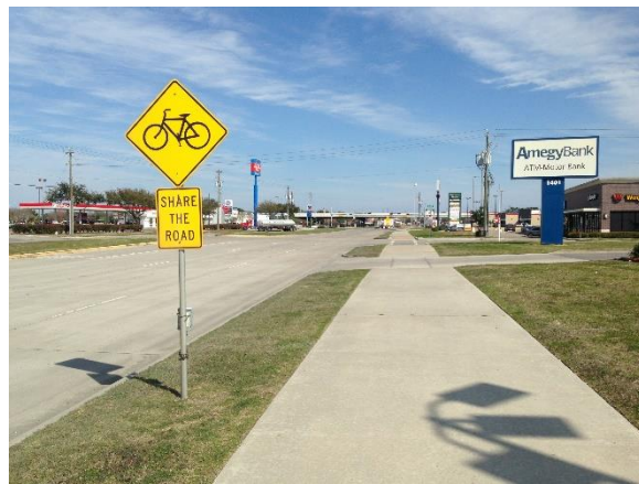
Image 6: Trail along Fairmont Parkway Facing East
