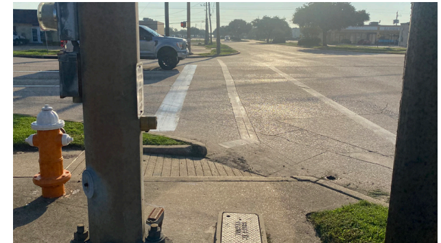
Utility infrastructure impeding pedestrian ramp and sidewalk Source: Halff
