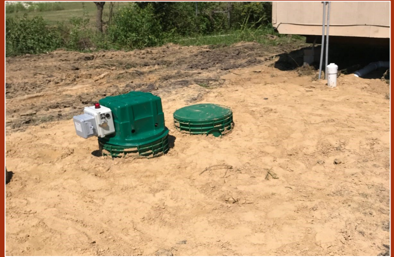
New aerobic OSSF
