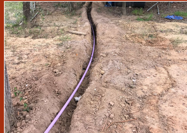
Installation of new spray field
