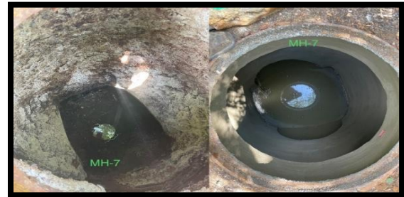
Figure 8. Manhole lining 8
