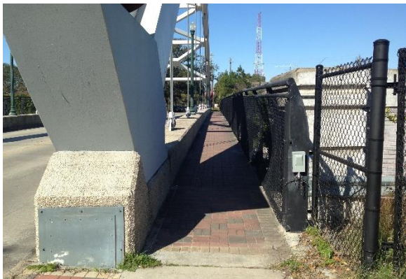
Image 19: Sidewalk along Graustark Street Northbound Facing North
