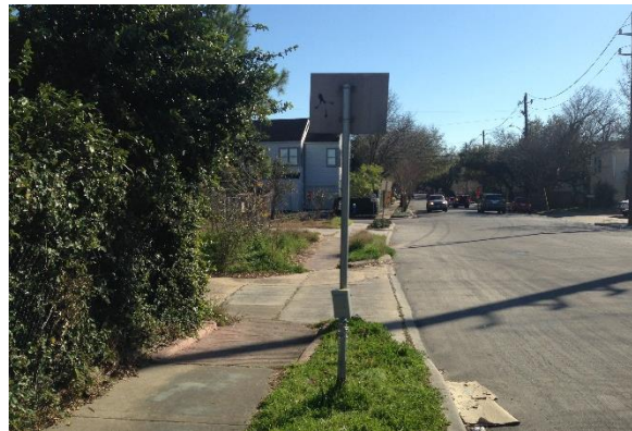
Image 4: Sidewalk along Hazard Street Northbound Facing South
