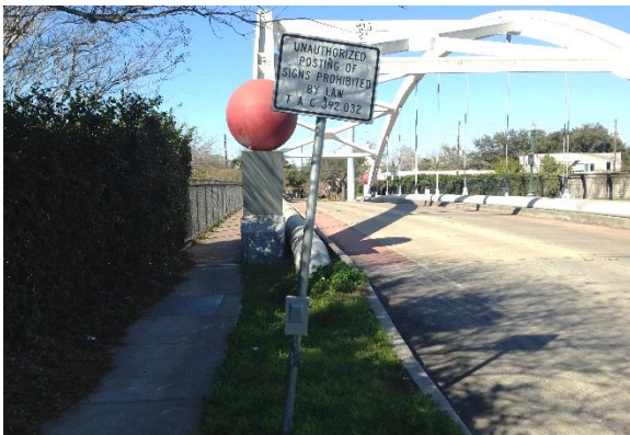
Image 1: Sidewalk along Hazard Street Southbound Facing North
