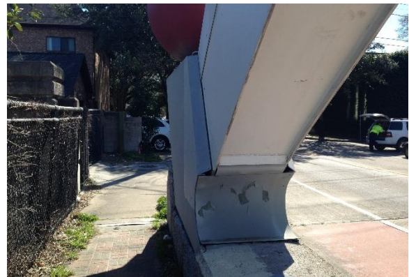
Image 16: Sidewalk along Mandell Street Northbound Facing South
