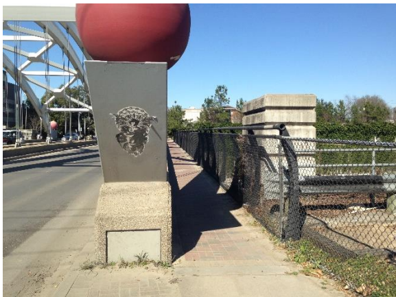
Image 23: Sidewalk along Montrose Boulevard Northbound Facing North
