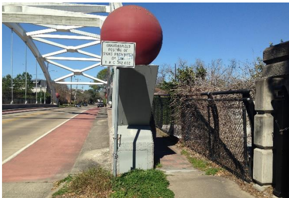
Image 15: Sidewalk along Mandell Street Northbound Facing North
