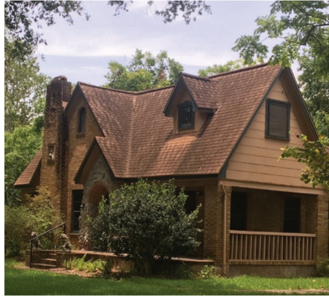
Existing Downtown Single-family Structure
