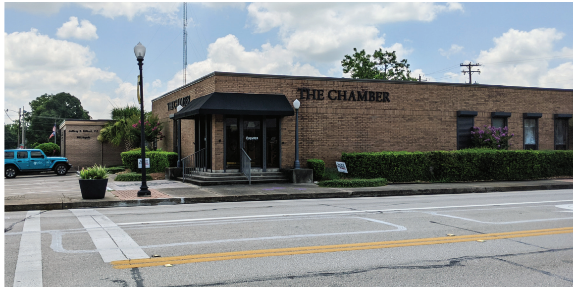
Existing Downtown Office - Chamber of Commerce
