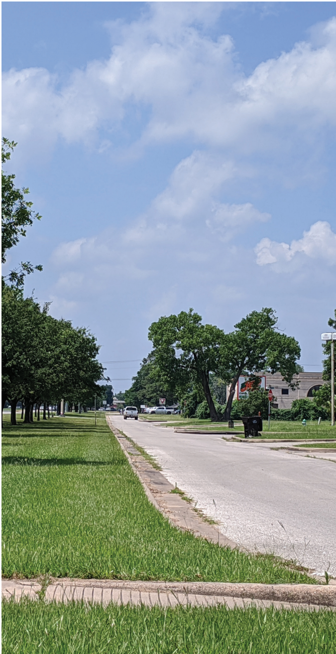
Existing Front Street Facing North
