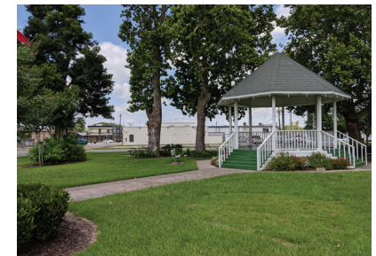
Existing Gazebo at Veterans Park
