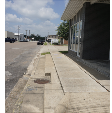
Existing High Sidewalk
