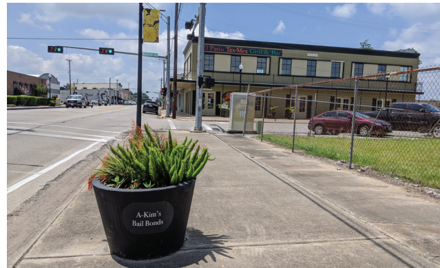
Existing Streetscape along Velasco Street
