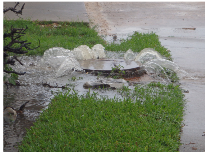
PHOTO: Sanitary Sewer Overflow
