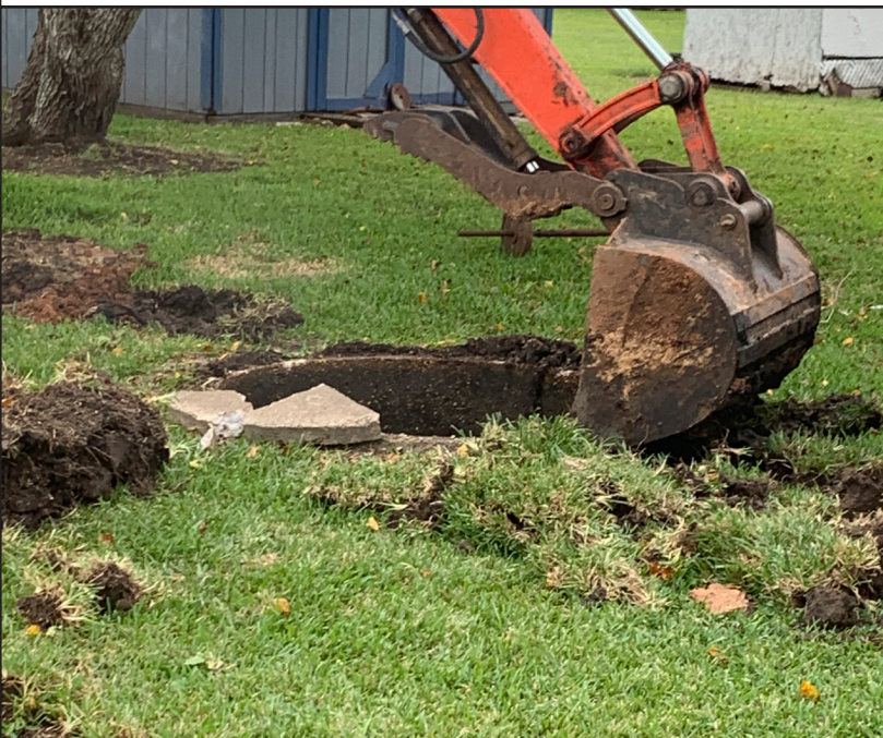
PHOTO: Decommissioning of a conventional septic system
