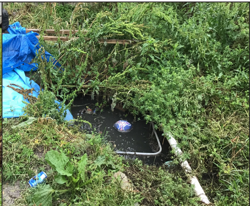
PHOTO: Surfacing sewage from a failed on-site sewage system
