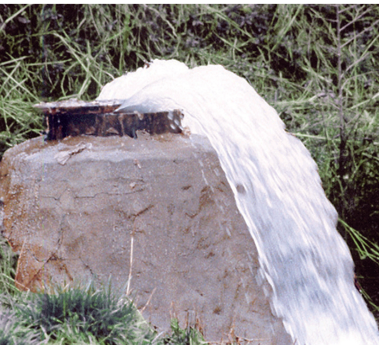
PHOTO: Sanitary Sewer Overflow
