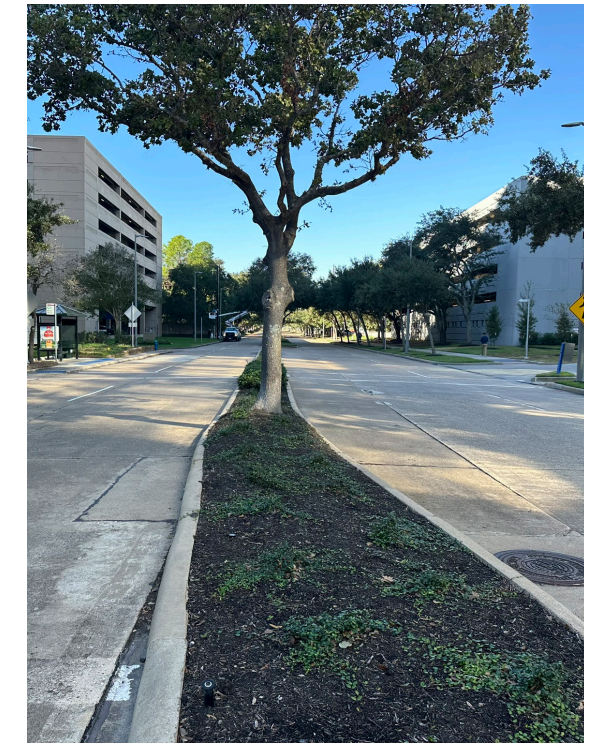
Grisby Road currently has curb and gutter drainage on a majority of the corridor
