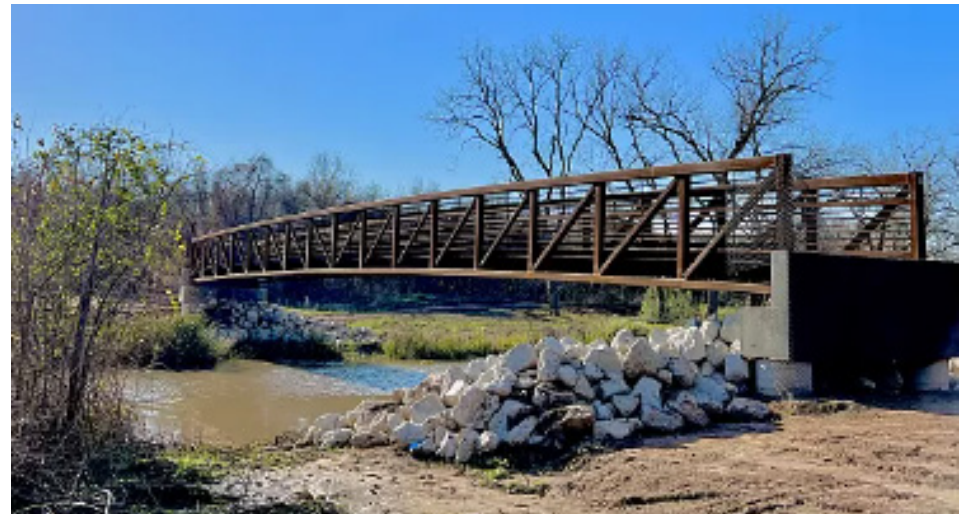
Existing pedestrian bridge in Sugar Land
