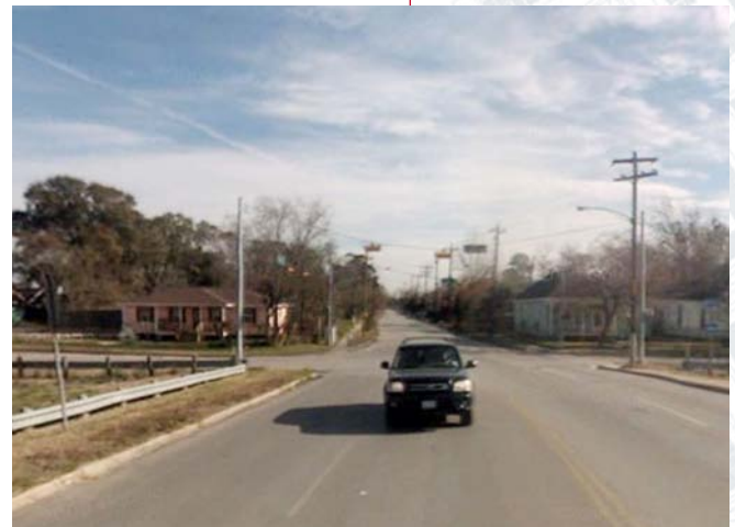
Western gateway at Quitman Street and Interstate 45
