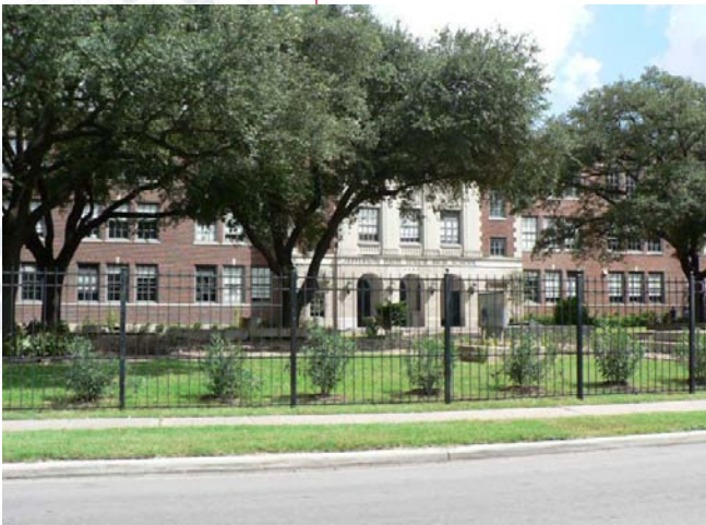
Existing Jefferson Davis High School.
