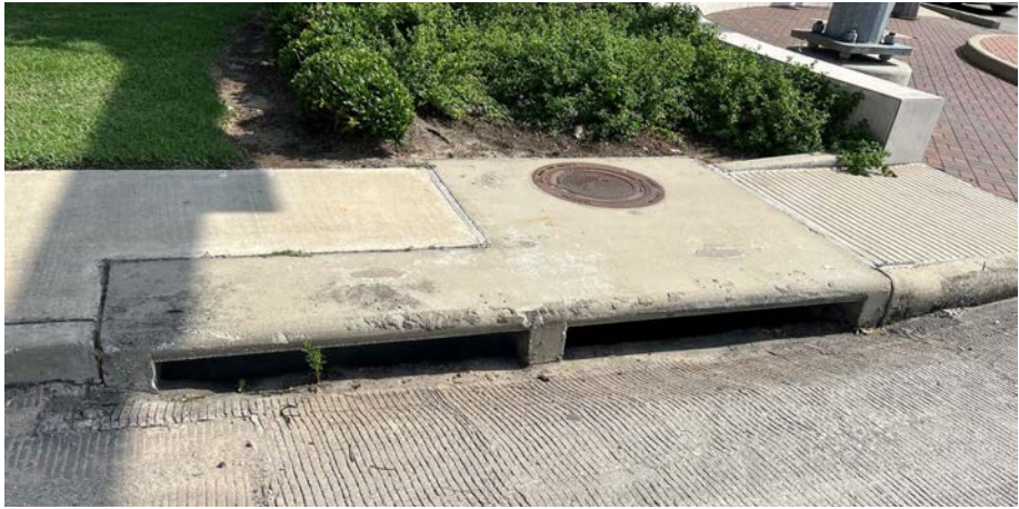
Figure 33: Curb Inlet
