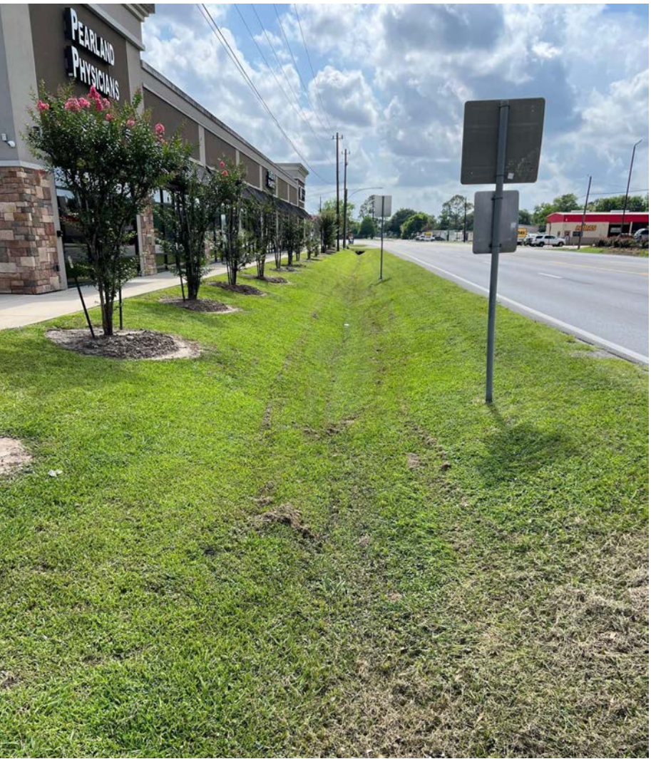
Figure 34: Open Drain
