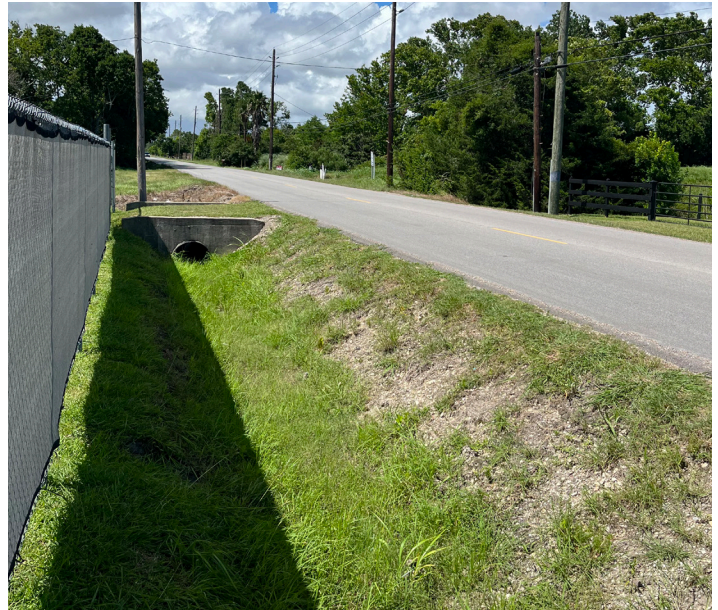
Open Ditch drainage along Cemetery Road
