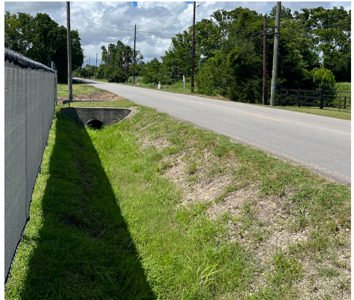
Open Ditch drainage along Cemetery Road
