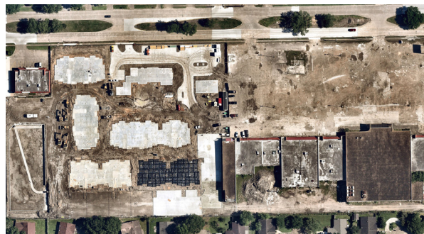
Construction of Edison Lofts, 2020
