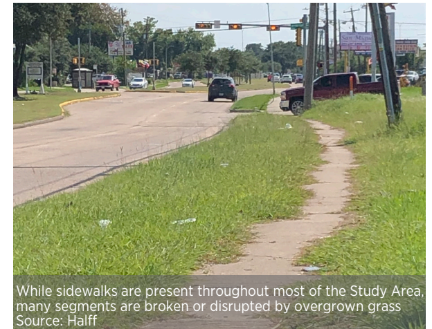
Discontinuous sidewalk segment along Fondren Rd. Source: Halff
