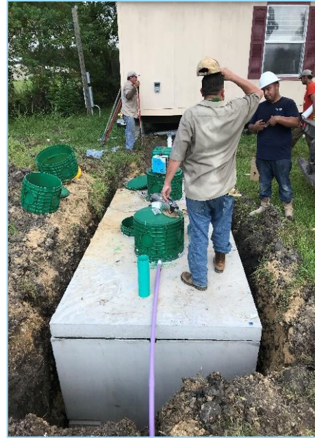
Figure 4. Septic tank replacement
