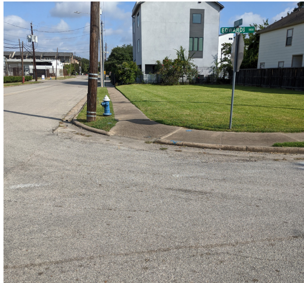
Diagonal Poor Ramp
