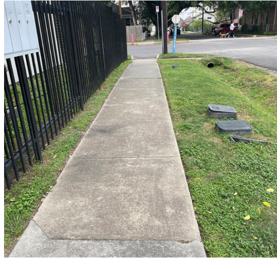
Condition B: Flat and less than 5 feet wide
