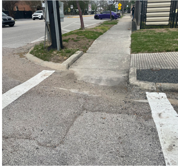
Directional Poor Ramp
