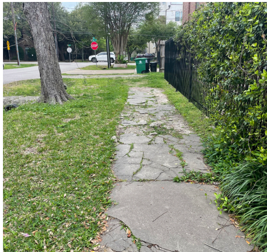
Condition D: Poor condition and less than 5 feet wide
