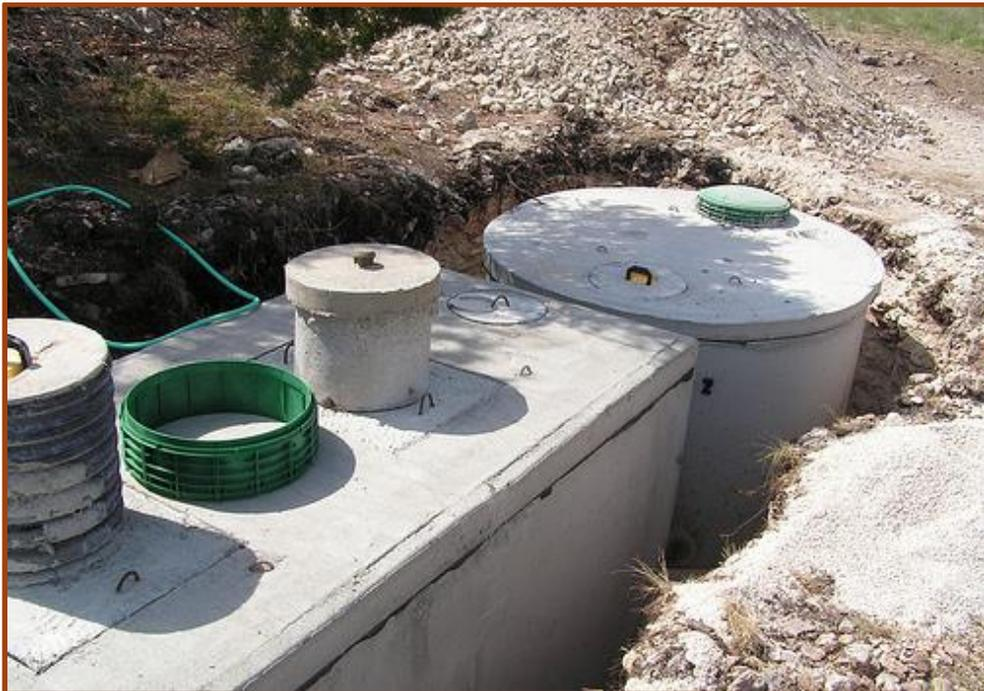
Figure 13 - Installation of an OSSF
