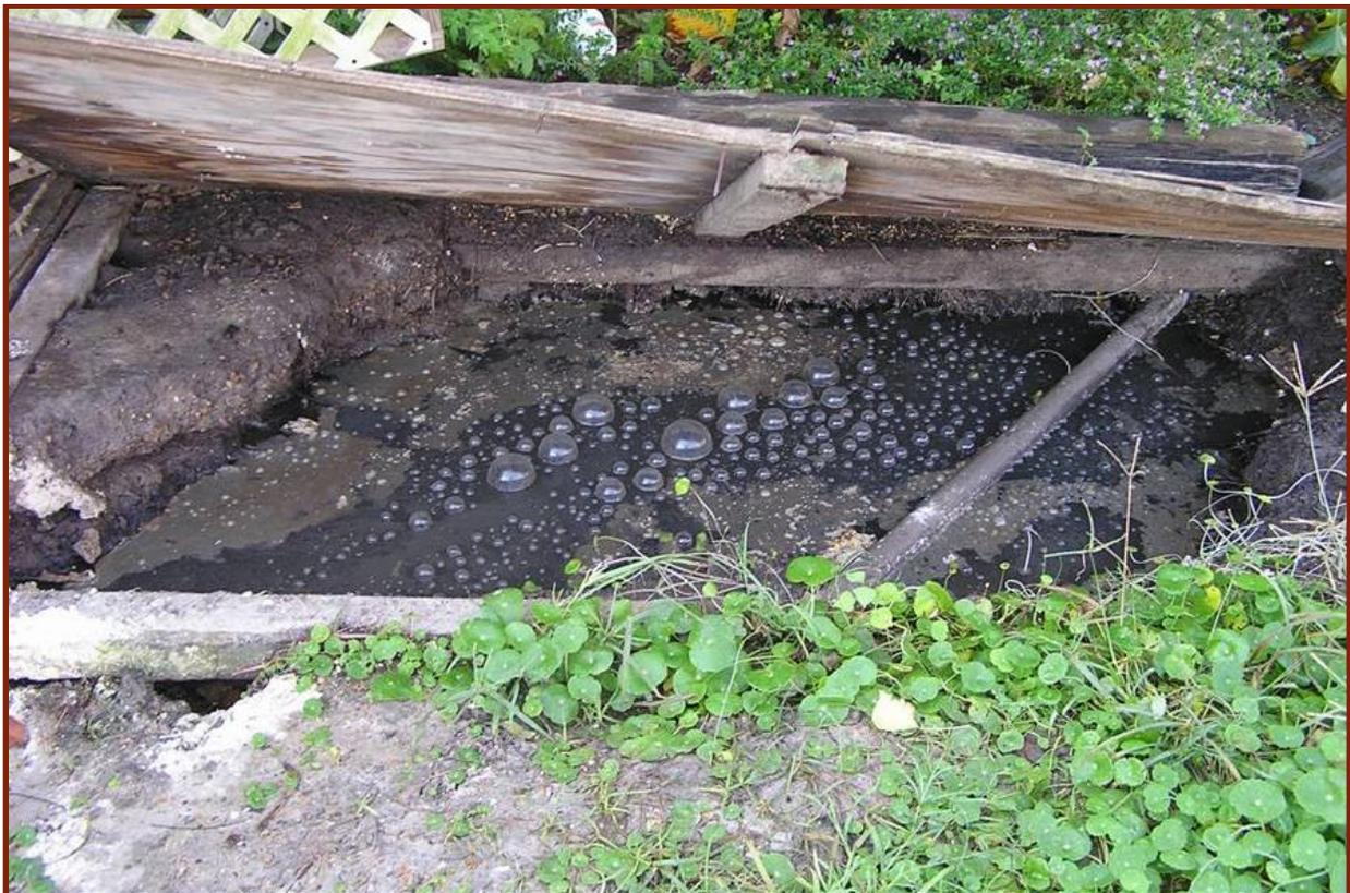
Figure 11 - Discharge from failing OSSF
